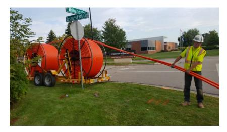
Teel conduit is being installed across Alliant's service area in Iowa and Wisconsin to improve its telecom network's security, speed, and reliability. For a utility with a large service area including more than 970,000 electric and 420,000 natural gas customers, reliability and capacity are is crucial during critical events. The conduit will protect the existing infrastructure and allow for later expansion of network capabilities while providing cost savings to Alliant Energy.
